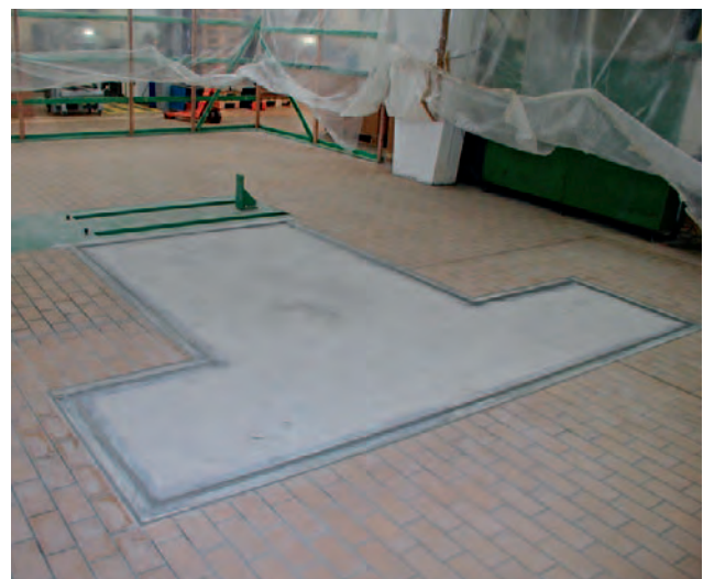
Cast foundation block
