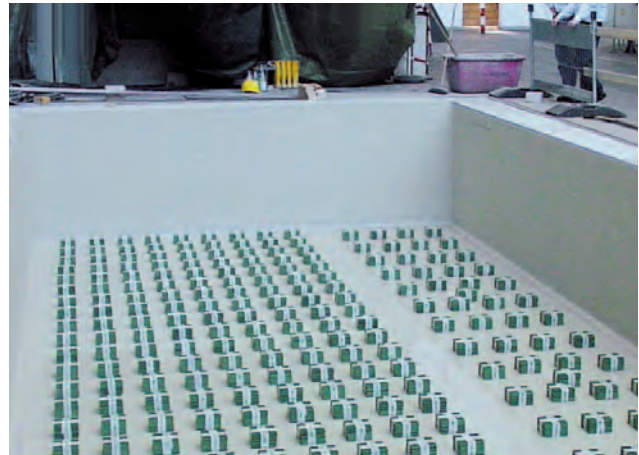
Foundation pit with Bilz isolation pads laid out
