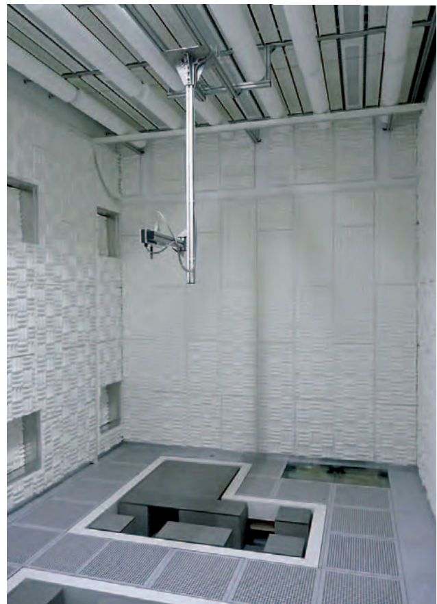
Experimentation room with 4.2 m clear room height and acoustic isolation materials (supplied and installed by Bilz). Source: Binnig and Rohrer Nanotechnology Center (IBM Research, Zurich).
